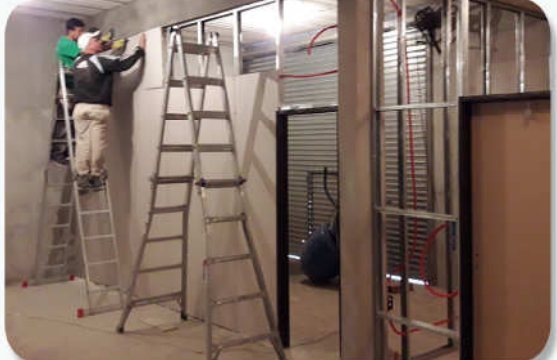
Some of the workers at the future church building
