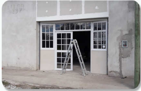
The church building is coming along
